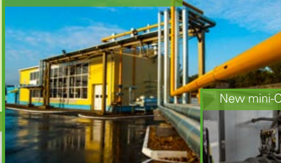
New CHP and boiler house
